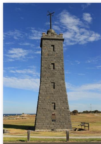
Williamstown Light-house more commonly known as the Williamstown Timeball Tower, is situated at Point Gellibrand, in the Melbourne suburb of Williamstown. The Williamstown tower was built in 1849 of local bluestone. It was originally a lighthouse, and later served as a timeball tower from 1861 to 1926.
