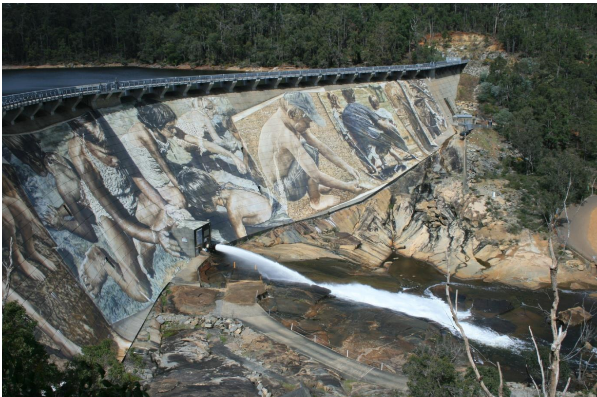
Wellington dam on the Collie River (photo Rory O'Brien)
